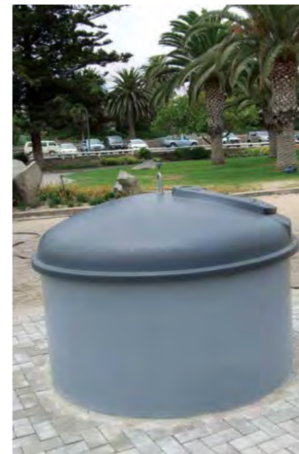
Recycling initiatives include the introduction of deep waste collection containers sunk vertically into the ground to a depth of five metres. Gravity helps to compress the waste, resulting in the need for less frequent emptying of the containers.
