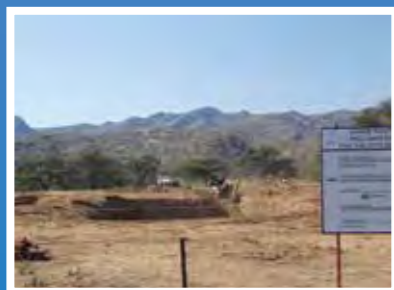
Construction of Ujams Wastewater Reclamation Plant commences
