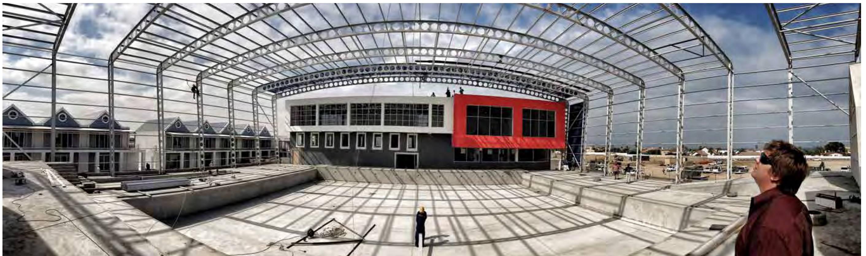
The new swimming pool complex in Swakopmund uses translucent polycarbonate sheeting that has never been used before in Namibia. With a span of 41 metres, the arch of the roof structure poses tough engineering challenges. Below, before the sheeting was applied and above, after.
