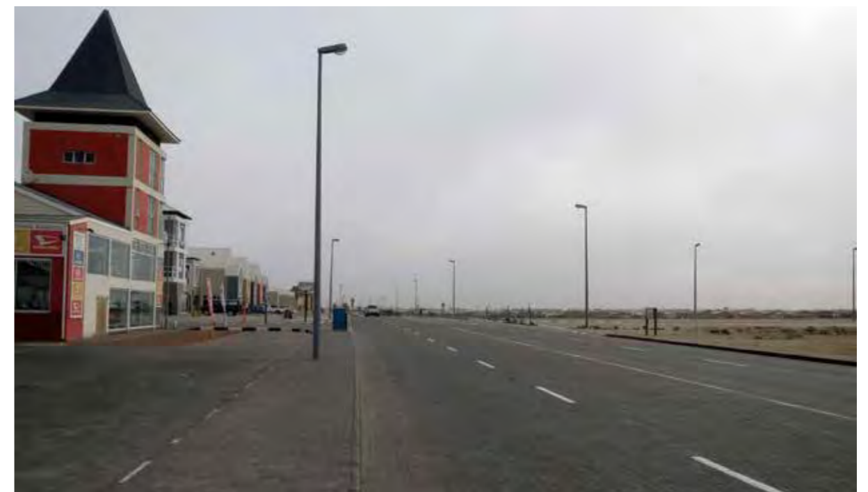
Interlocking bricks are used for resurfacing of some roads in Swakopmund.
