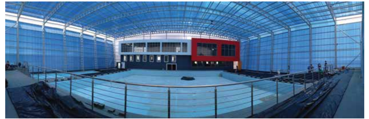
The new swimming pool complex in Swakopmund uses translucent polycarbonate sheeting that has never been used before in Namibia. With a span of 41 metres, the arch of the roof structure poses tough engineering challenges. Below, before the sheeting was applied and above, after.
