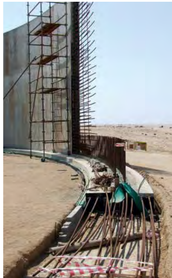
Part of the new sewerage works.
