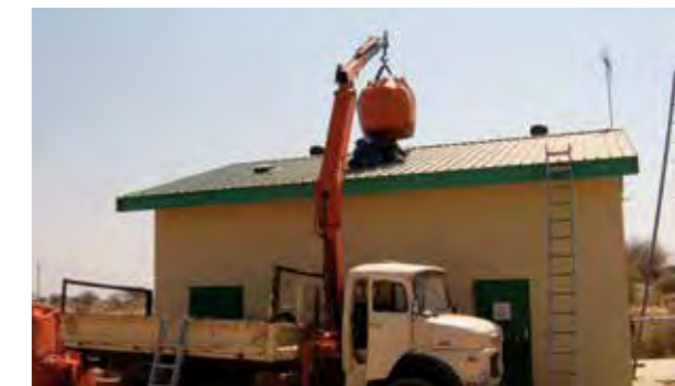
Loading of Granular Activated Carbon through the roof into a carbon filter inside the building.
